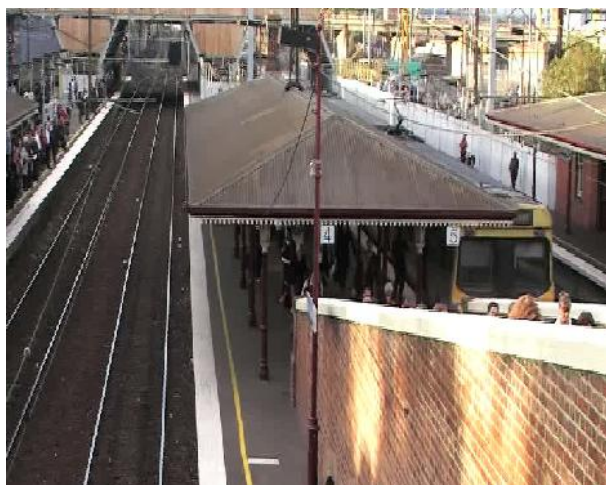
Figure 5: Observed conditions at North Melbourne Station
